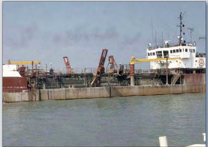
Dredge operation in Toledo Harbor.
